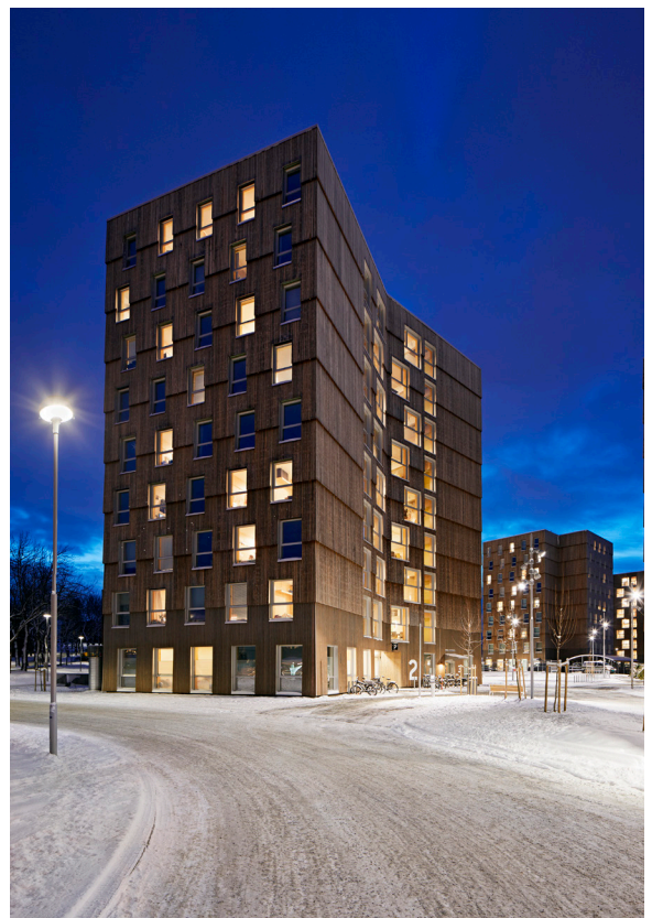
Moholt student apartments - photo Ivan Brodey
